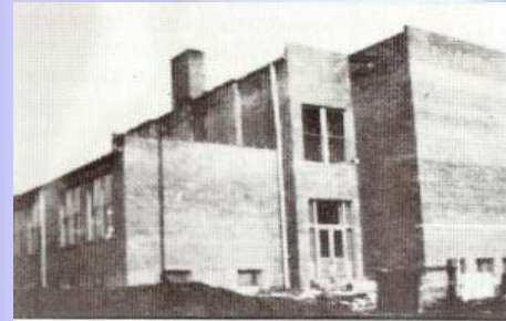
Bethel Township School before the tornado.
