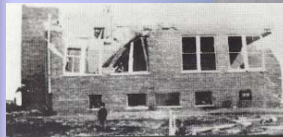
Bethel Township School after the tornado.
